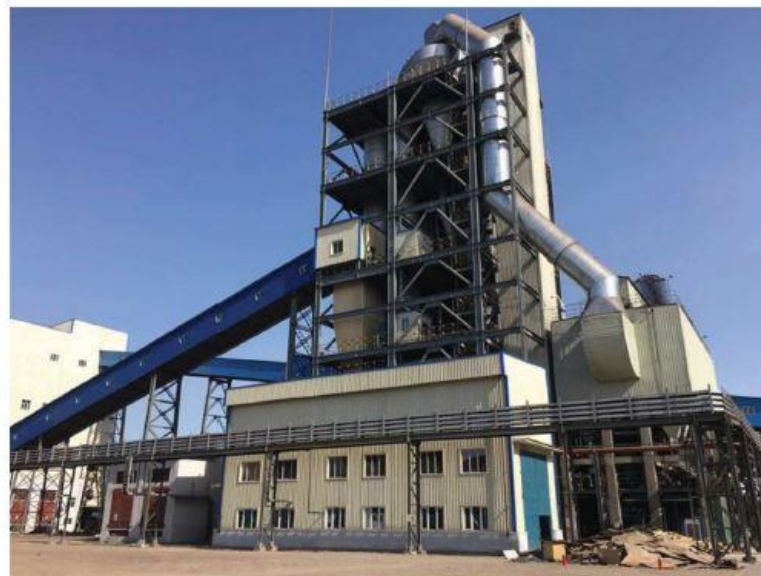
Figure 6. Industrial suspension magnetization roasting system with a throughput of 1.65 million t/a for beneficiation of specularite ore in JISCO.
